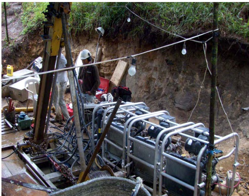
Figure 10.1: Hydracore Series III rig drilling hole LA-38
