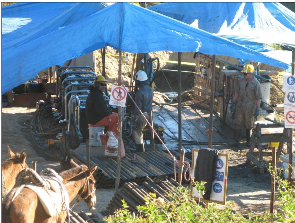
Figure 10.1 Drill Rig at Romero
