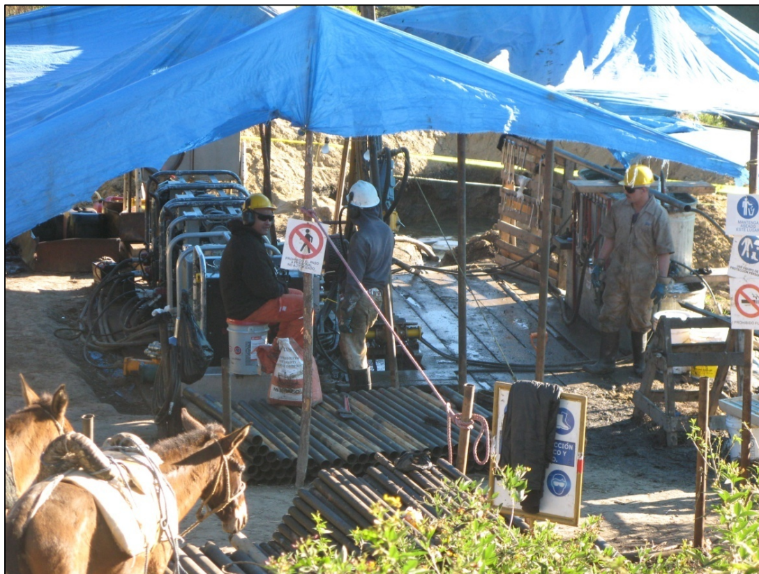
Figure 10.1: Drill Rig at Romero
